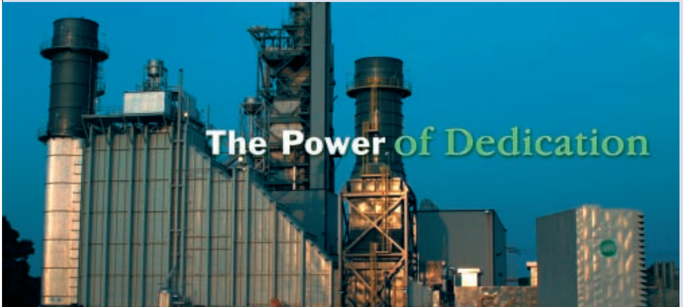
Thomas B. Fitzhugh Generating Station
